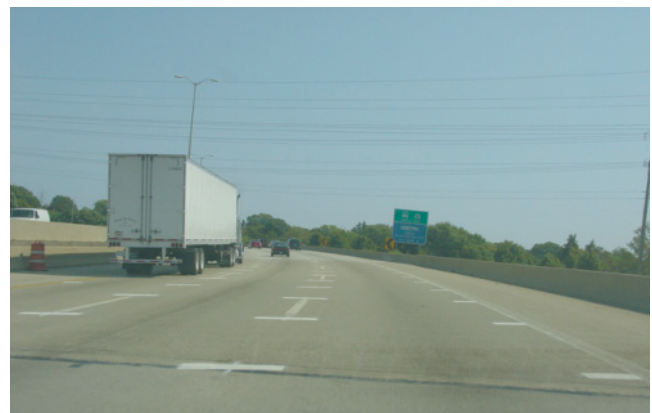
FIGURE 2 Experimental transverse pavement marking treatment.
