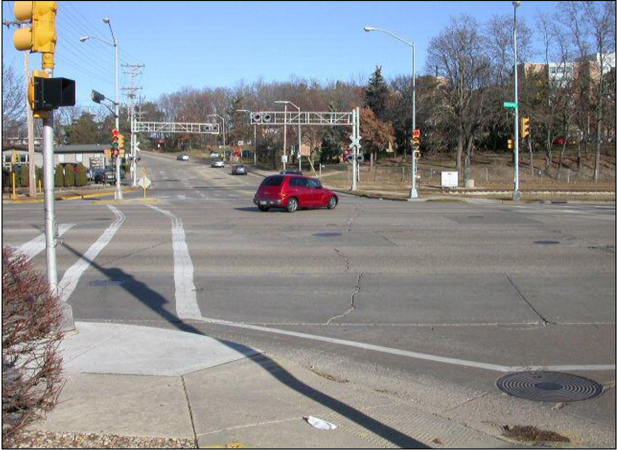
FIGURE 8 Farley Avenue at University Avenue, Madison WI.
