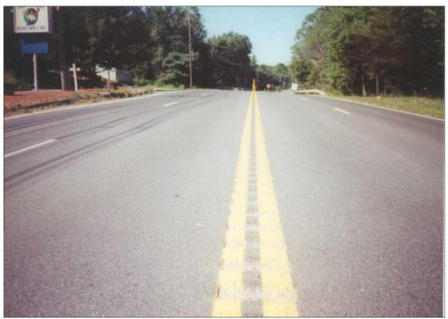
FIGURE 1 Centerline Rumble Strip on State Route 20 in Massachusetts.
