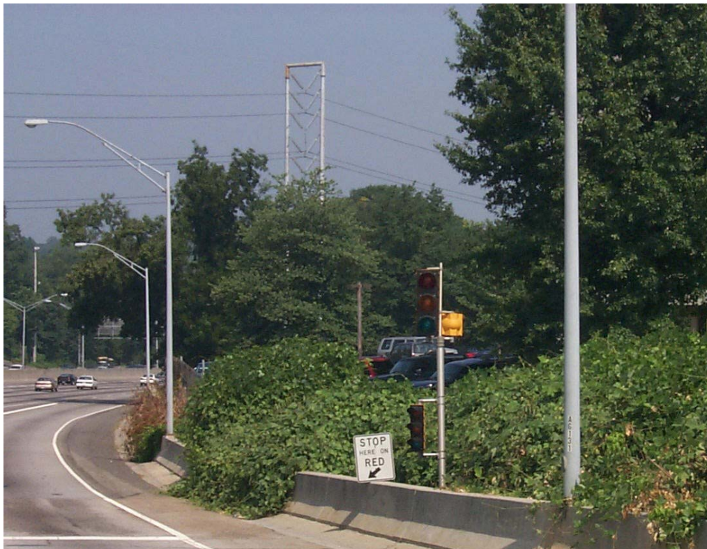
Figure 7-1: Ramp Metering Signals
